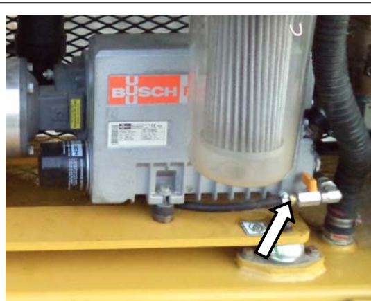
Drain hoses are operated by hand valve. 049-42-55-001B
